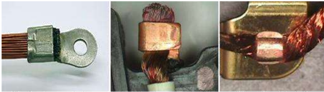
▲Fusing of covered wires
